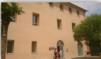
Façana principal de Can Tirel
